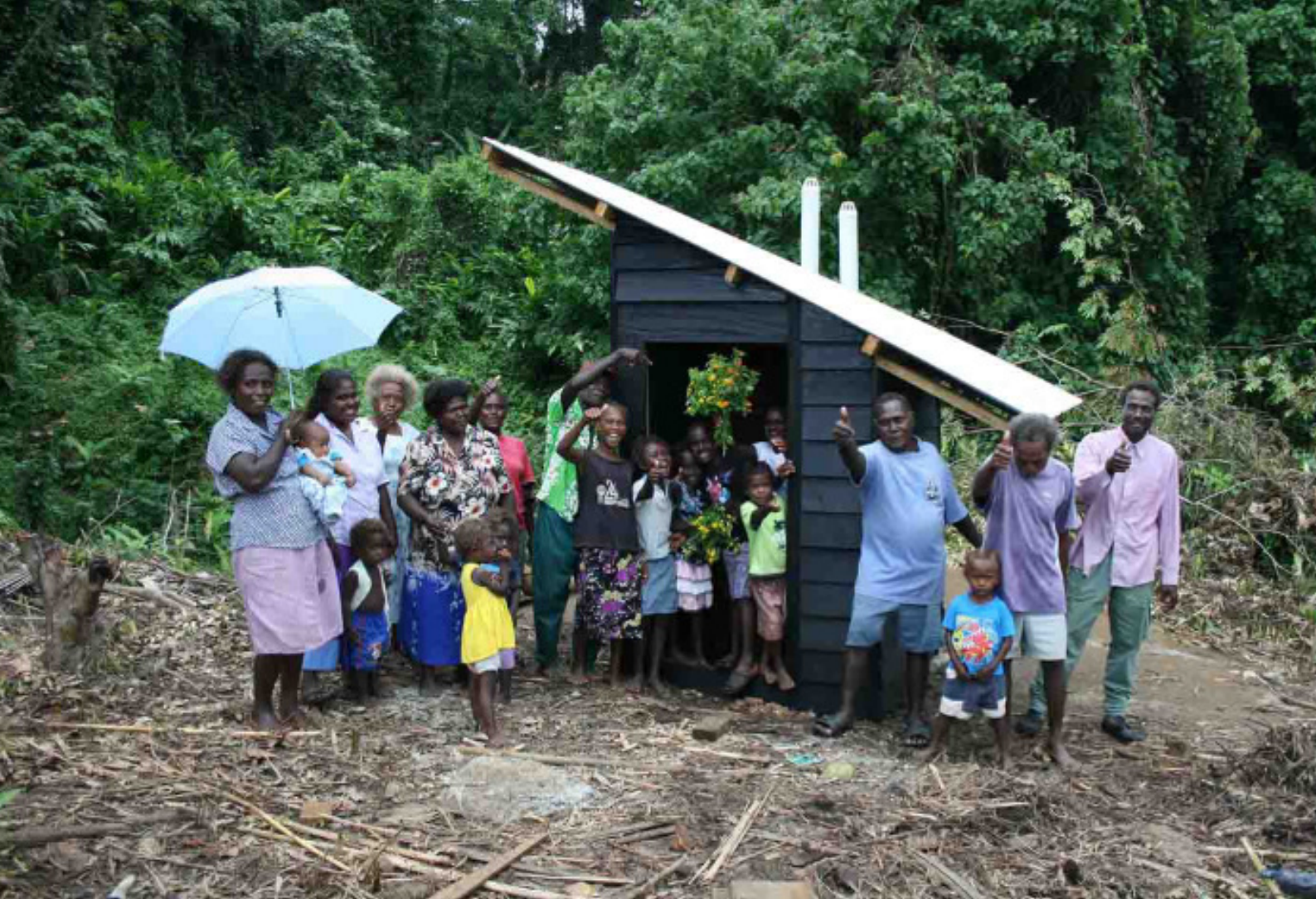
New Latrine in Keigold, Ranongga, Solomon Islands Built by Emergency Architects Australia and the Community of Keigold
